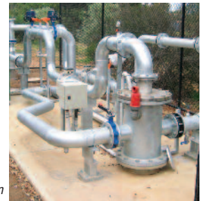
Submersible pump installation
