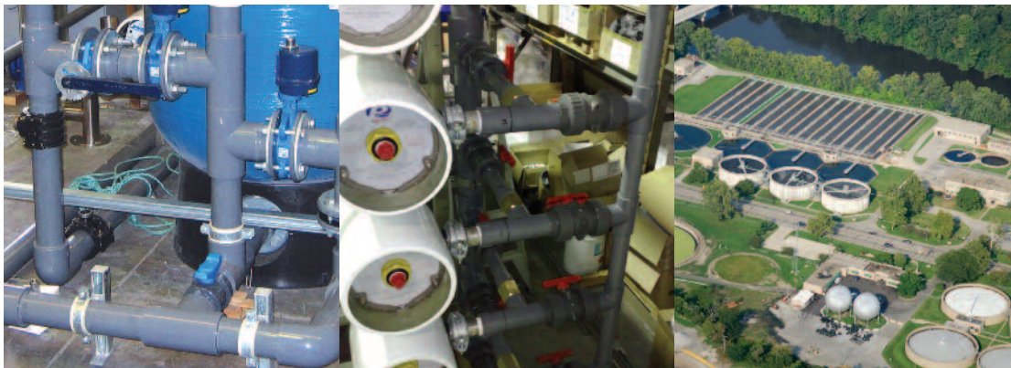
Maric valves control backwash flow rate in a media filter
